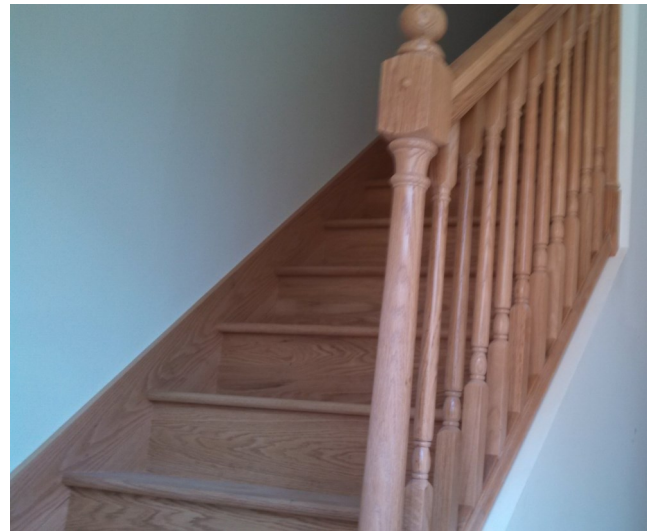
Stained oak treads/risers/skirtboard with stained oak railing
